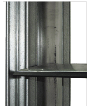
Torn aluminum jamb seals obstructing blade operation
