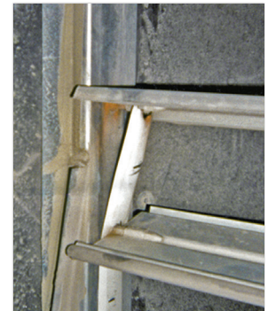
Torn aluminum jamb seals obstructing blade operation
