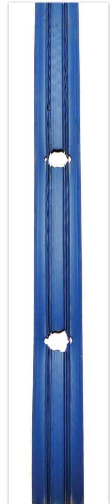
Appearance of frame seal after 96 months
